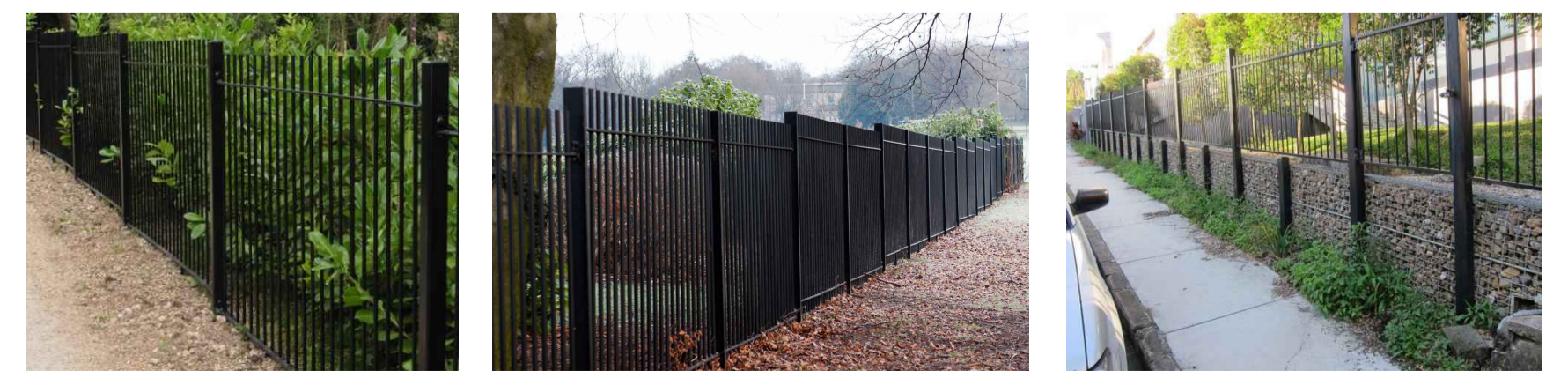
A 1.2m high galvanised steel fence B 2.0m high galvanised steel fence C Galvanised steel fence on gabion wall (overall height 2.0m)
