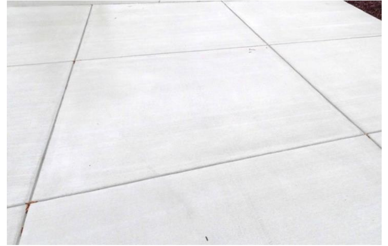
Cast In-situ Concrete Surface
